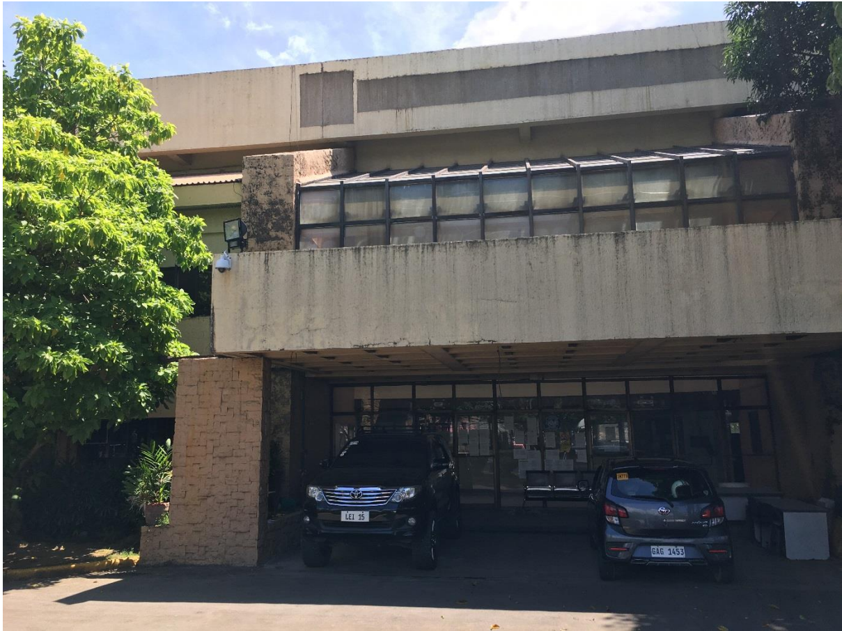
Front View of old MEZ Admin Building
