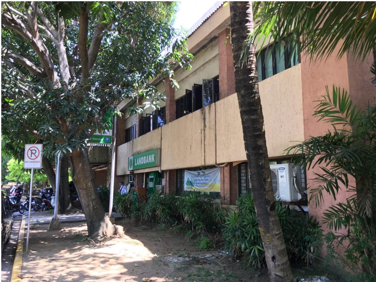
Front view – A portion of the ground floor occupied by Landbank
