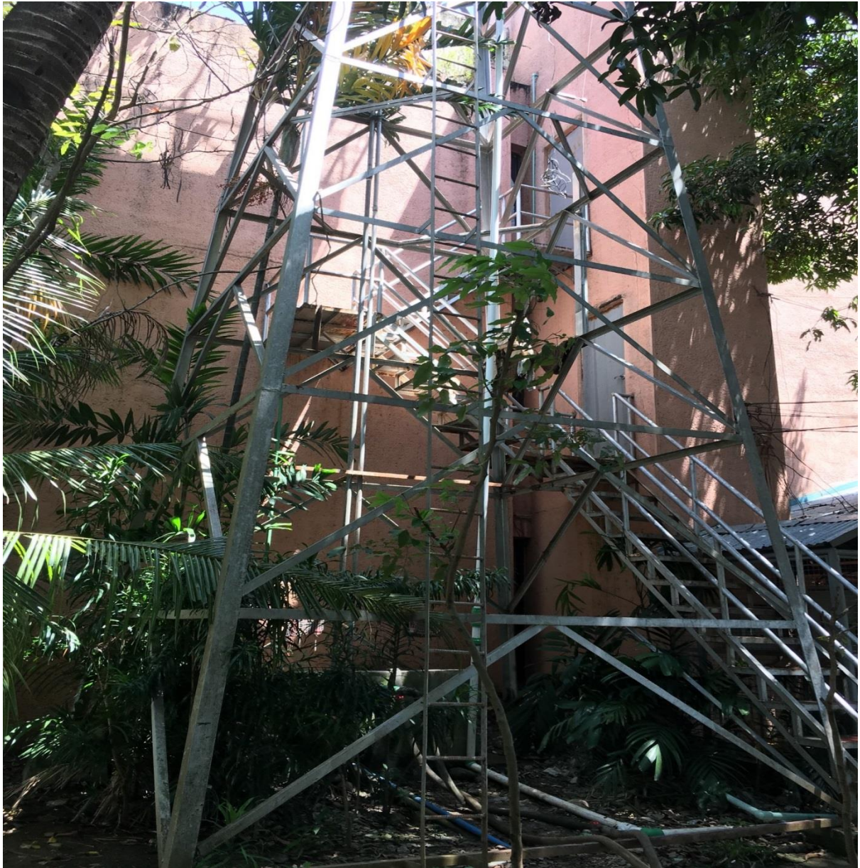
Right View of old MEZ Admin Building
