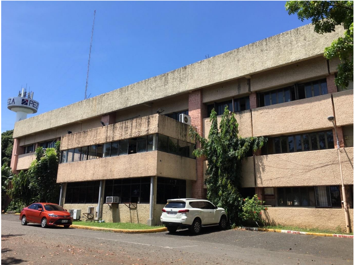
Rear View of Old MEZ Admin Building
