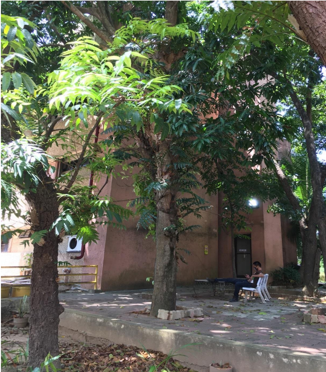
Left View of old MEZ Admin Building
