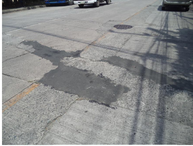
South Avenue (near Daiki OM )
