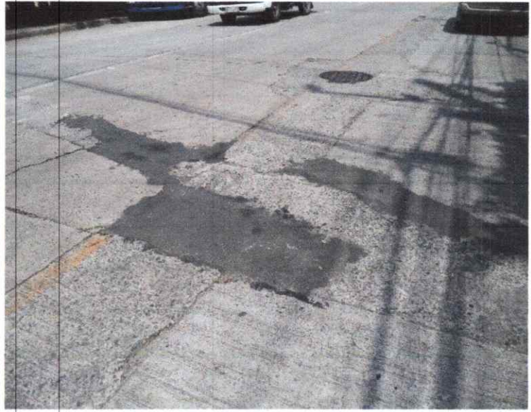
South Avenue (near Daiki OM )
