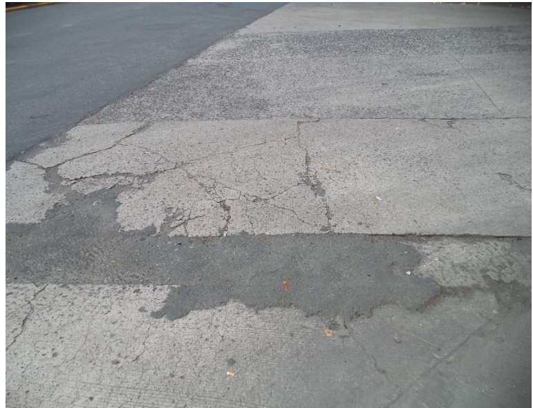
Road E (near Hitec RCD), A=75.60 m2
