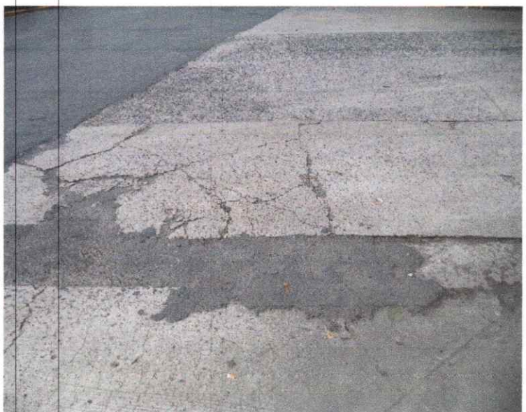
Road E (near Hitec RCD), A=75.60 m2
